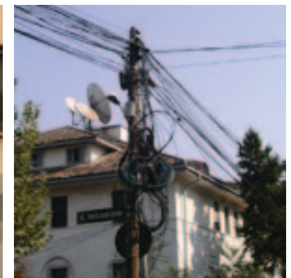
Fig. 9. Suspended wirings
