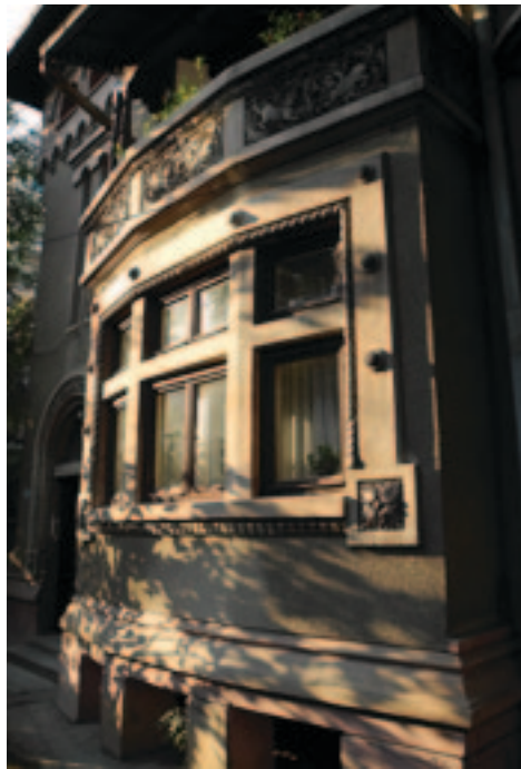
Fig.18. The façade has been enriched by the juxtaposition of contrasting surfaces: the rough render, the smooth cornices and moldings and the chiaroscuro of the cast stone elements.
