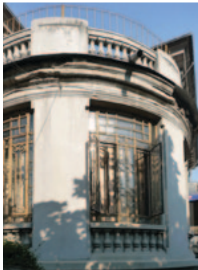
Fig. 6. The technical design solutions identified in the district exhibit an enviable variety, the image shows an external grill integrated with a glass frame to form a second window.
