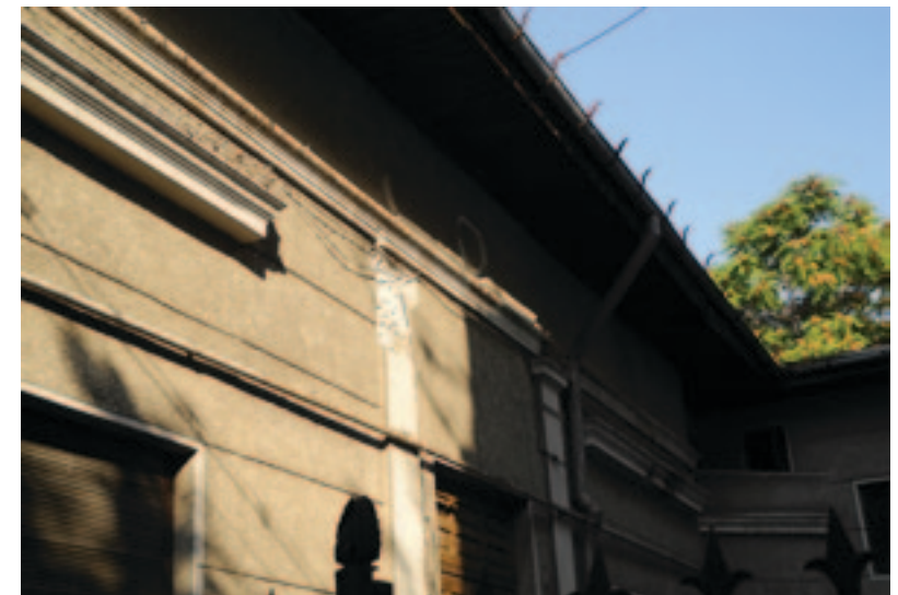
Fig.17. The artificial stone capital has been lost and the restoration of the façade requires to make a replica, preferably casting a mould of the remaining capital.
