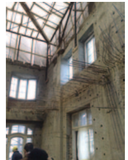
Fig.3.12. Peripheral load bearing tube in reinforced concrete
