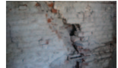
Fig.3.4. Crack in inner wall
