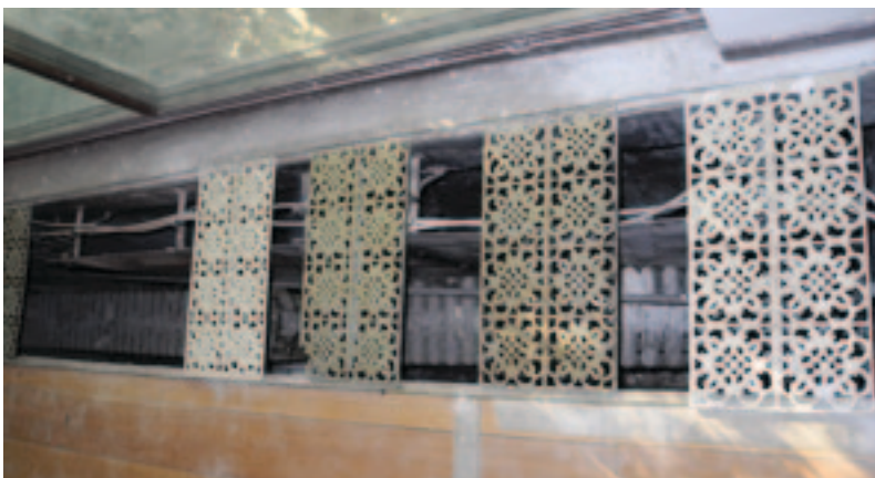
Fig. 7. The heating system of the building, located under the floor in correspondence of the fixtures and hidden by refined cast iron grids.
