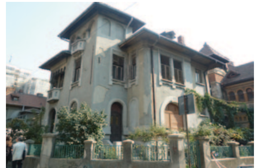
Fig. 3. Bucharest, modernist borough. An example of a villa in picturesque style with conservation problems in the outer plasters (Photo R. Picone 2011)
