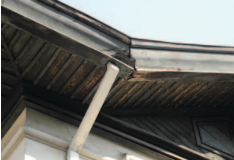
Fig. 5. The wooden intrados of the eaves of a building. The leakage of the drainage system, hidden in the cornice, has caused the strong decay of this part of the roofing.
