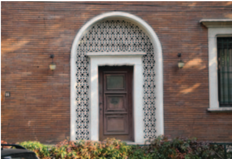
Fig.11. The main door of the building of Strada Atena 14. The brick facing, made by very thin elements and relatively thin joins, contrasts with the marble framing, of a rather classical style, of the openings. Exceptionally fine is the marble grid around the entrance door.
