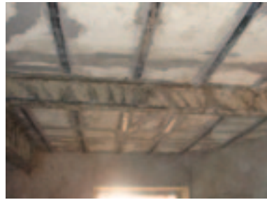
Fig.2.11. Strengthening of RC floors with carbon fiber strips and fabrics
