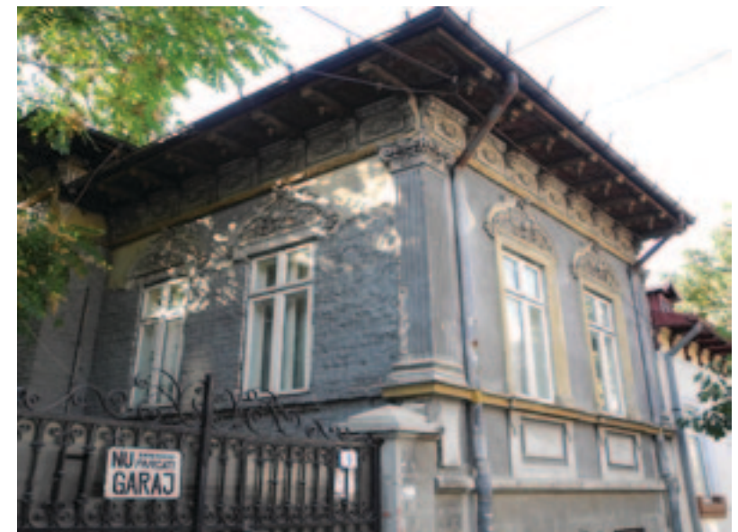
Fig. 18. Some works in progress show a lack of attention for the conservation of plasters and important decorative parts. After extensive demolitions and rebuilding, they often chose colours that are entirely foreign to the original characteristics of the buildings.
