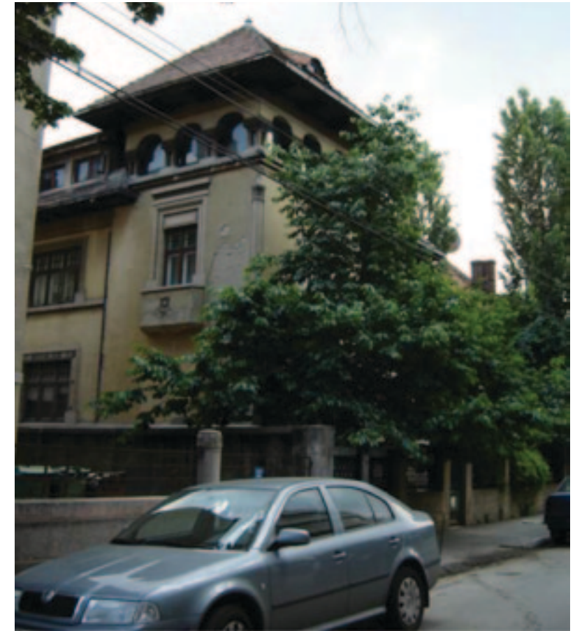
Fig. 6. Smooth plaster with moderate presence of missing areas. The general good state of preservation of the original plaster can be noticed. Roofing with projecting eaves.
