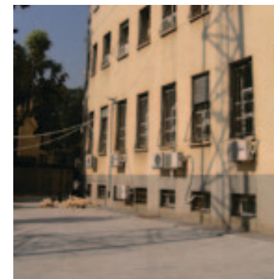
Fig. 8. Additions altering the original appearance of the facade
