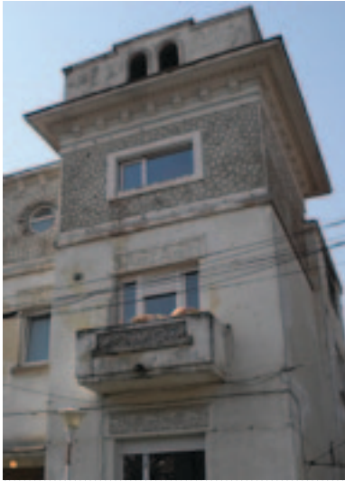
Fig. 21. The rare plaster of the upper level of this building, made putting on a rough render many flashing big quantities of mortar, then flattened, with the final effect of a series of irregular flat circular shapes on a rough bottom. This upper part of the façade and the above protruding eave, a classical cornice with even dentils, has a strong contrast with the lower, smooth, part of the façade.
