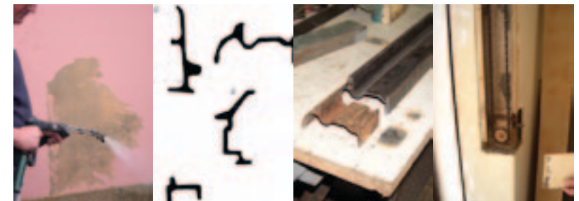
Alvaro Siza’s recent conservation project for Casa de Serralves, an Art Deco detached house in a Modernist neighbourhood of Oporto, proposed to maximise the preservation of the existing building through a ‘surgical’ intervention, namely on the exterior plasters, windows and technical devices which are preserved with local and accurate reparations. (Photos kindly provided by A.O.F.- Filipe Ferreira.)
