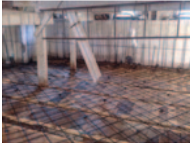
Fig.2.10. Steel mesh for reinforced concrete topping on wood floor
