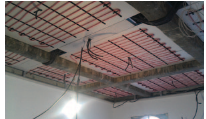
Fig.2.9. New heating and cooling equipment attached to the floors
