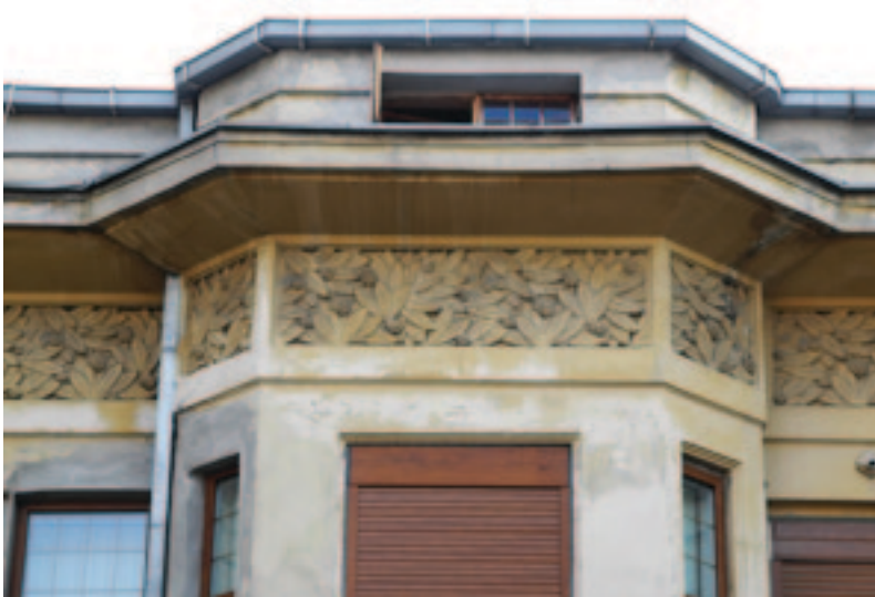
Fig.15. The refined flower motif in cast stone placed as a frieze at the top of the building, in correspondence of a bow-window. The chiaroscuro of these elements contrast with the flat plastered surfaces of the rest of the façade.
