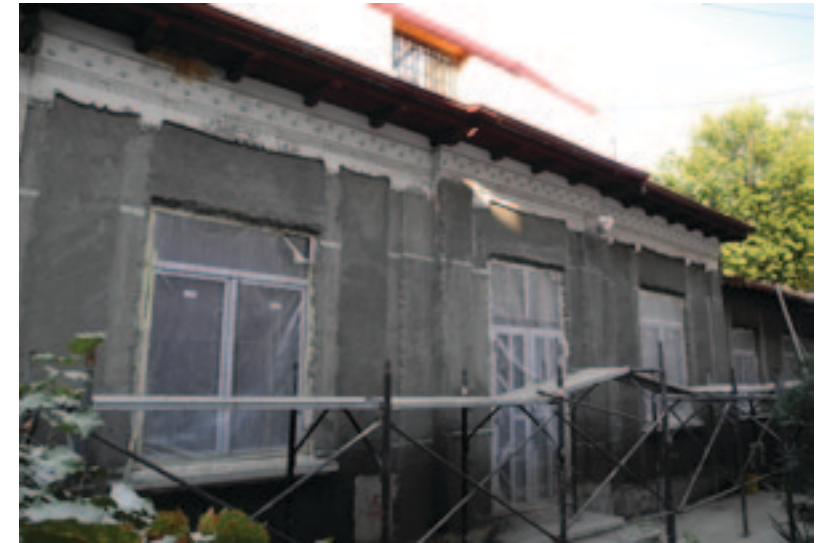
Fig.16. In the intervention, the plaster has been removed and only the relief decorated elements have been preserved.
