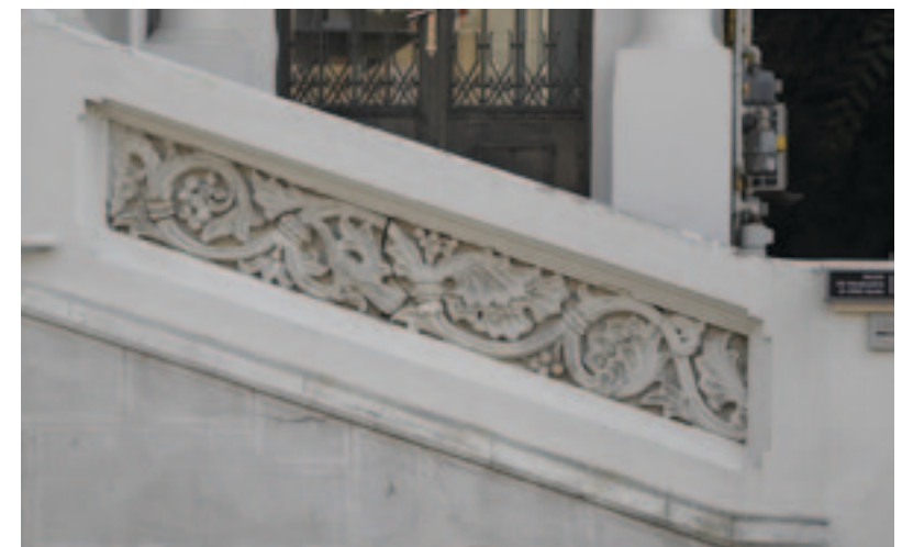
Fig.14. The cast stone decorating a stair parapet, over a wall in false ashlars.
