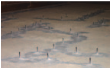
Fig.4.4. Grouting with epoxy resins at reinforced concrete slabs
