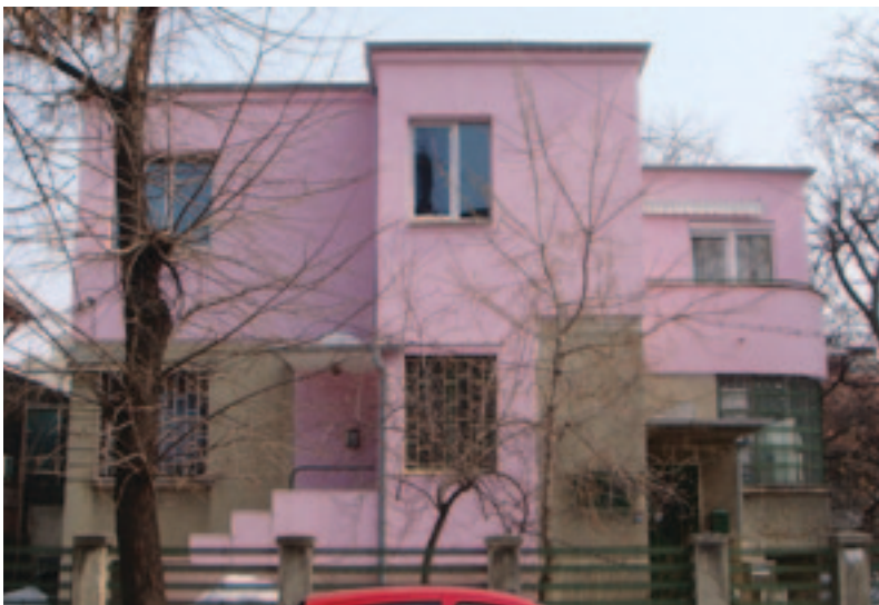
Fig.2. Thermal rehabilitation on Londra St: polystyrene and pink paint on façades.
