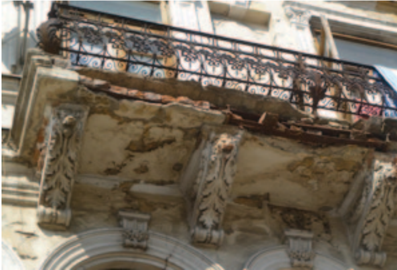
Fig. 2 Balcony in artificial stone shows its tough metal
