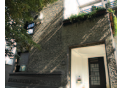
Fig. 23. The irregular shadowing of the surface given by a render only partially flattened.
