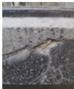
Fig. 27. Detail of the terrazzo cladding of the low fence wall of the building.
