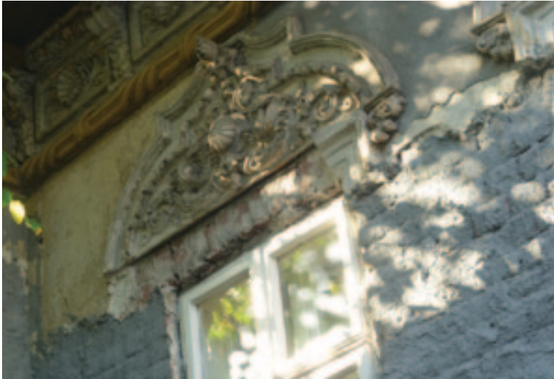
Fig. 4. An example of the decorative works in formats out of the molds and then mounted on the façade.
