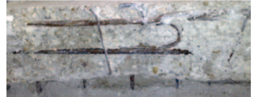
Fig.2.7. Exposed reinforcing bars at slabs and beams
