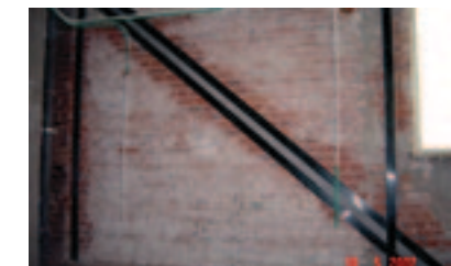
Fig.4.7. Strengthening of masonry walls with carbon fiber strips
