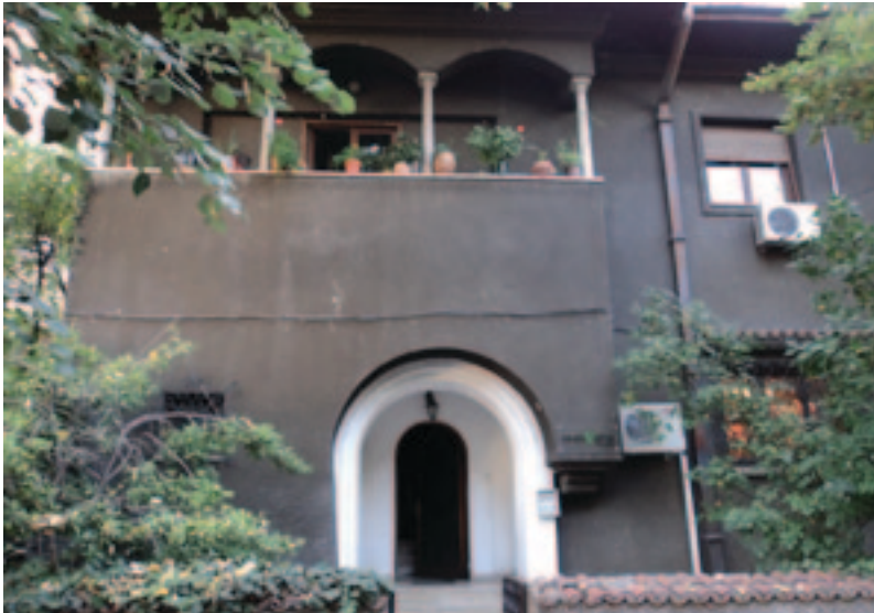
Fig. 9. Replacement of the façade finish, with a new gray one; interpretation of the image different from the original.
