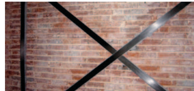
Fig.4.8. Strengthening of masonry walls with carbon fiber strips
