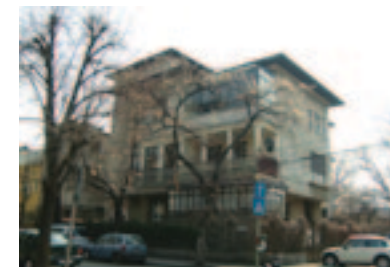
Fig. 26. Overbuilt structures on balconies in Strada Washington.
