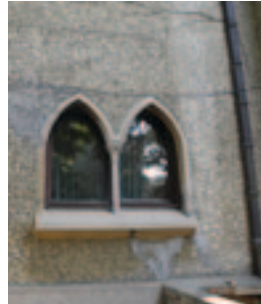
Fig. 25. The lack has been “repaired” with an improper mortar, damaging in an irreparable way the façade.
