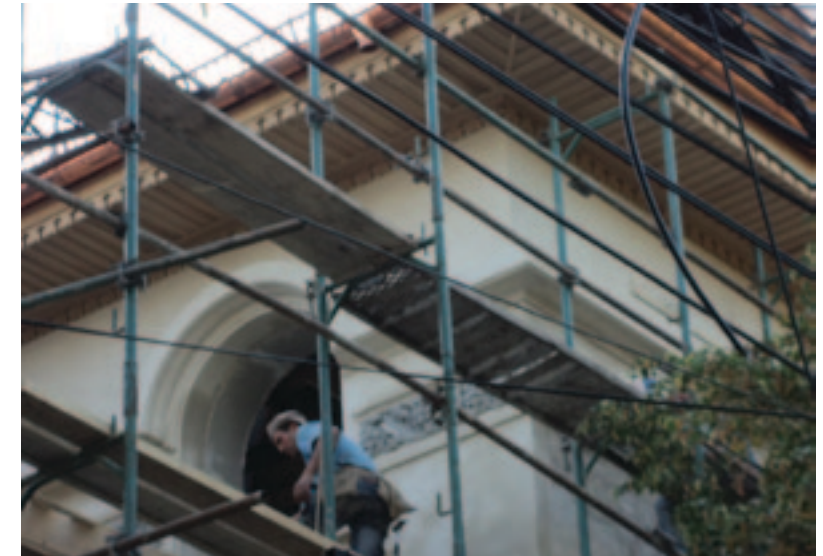
Fig. 4. Reproduction of original moldings.
