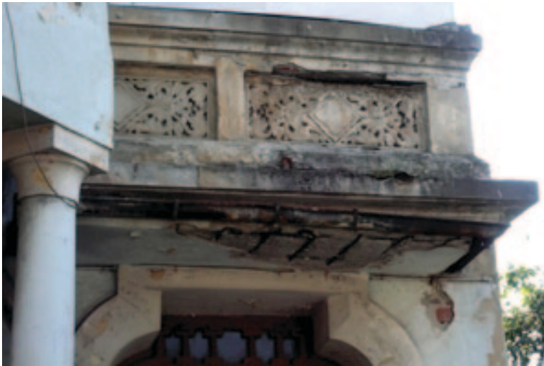
Figs. 6. Insertions in reinforced concrete. Phenomena of concrete cover detachment and oxidation of reinforcement bars.
