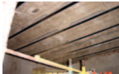
Fig.4.5. Strengthening of reinforced concrete beams with carbon fiber strips
