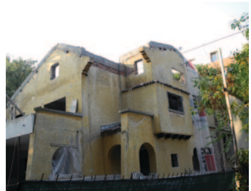
Fig.30. The kind of works made on this building, in particular the concrete curb at the top of the walls, makes it impossible to preserve the original fine plaster. The building, at the end of the works, will have a quite different aspect from its initial status, thus contributing to decrease the variety, and hence the richness, of this part of the town.
