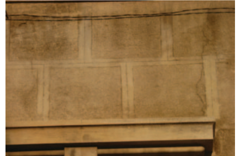
Fig. 3. Plaster shaped in imitation of stone.
